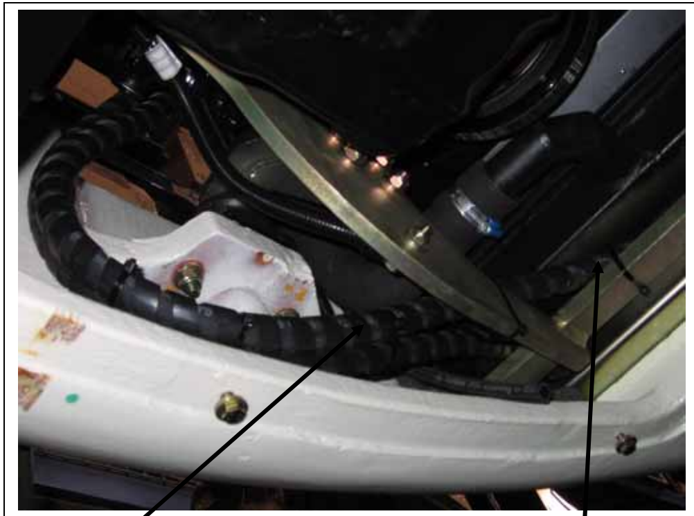
13/32" hose going into radiator compartment through an existing grommet.
